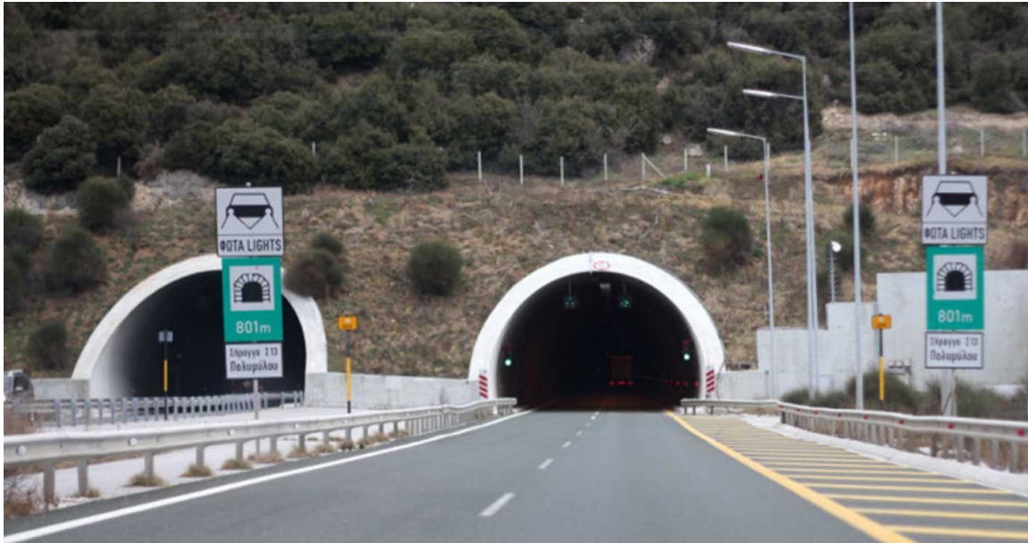
Figure 20: Polymilos tunnels (S13 tunnels) of Egnatia Motorway.
